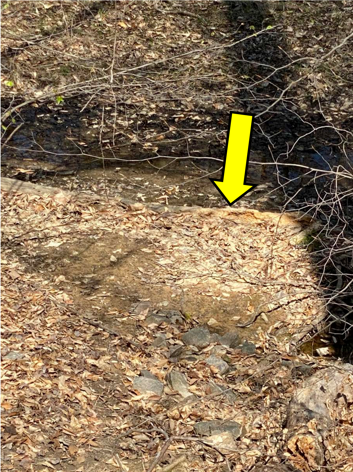
OF-11 (Photo 2 of 2) – Sediment deposition along creek bed downstream of outfall.
